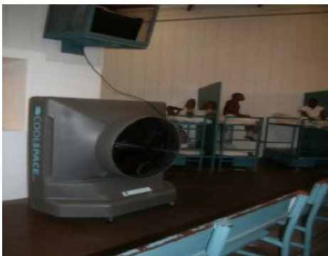
Cooling equipment employs a large fan inside about a 6-foot-by-6-foot box
